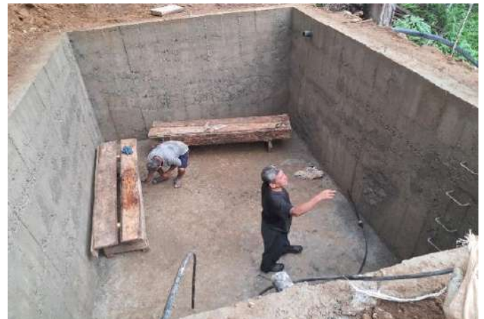
Reservoir tank construction
